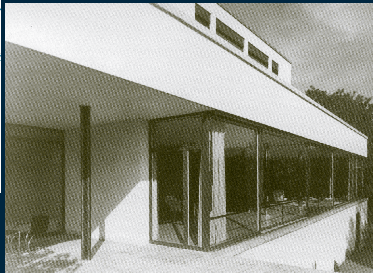
Tugendhat House Glass facade overlooking the garden
